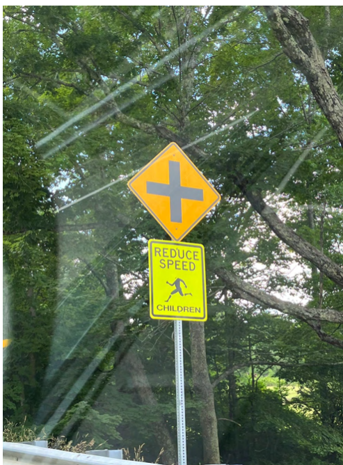
Example of a sign warning of an upcoming intersection and calling for speed reduction (Chesterfield, MA)
