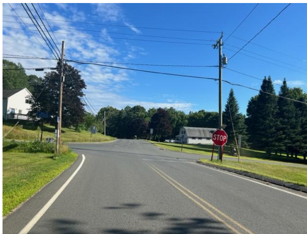
Intersection of North Rd and Easthampton/Kings Highway
