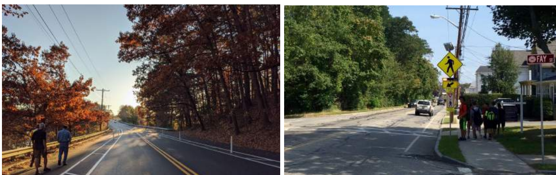
(Left) Flex-post protected walkway in Natick, MA (Right): Rectangular Rapid Flashing Beacon (RRFB) in Westborough, MA
