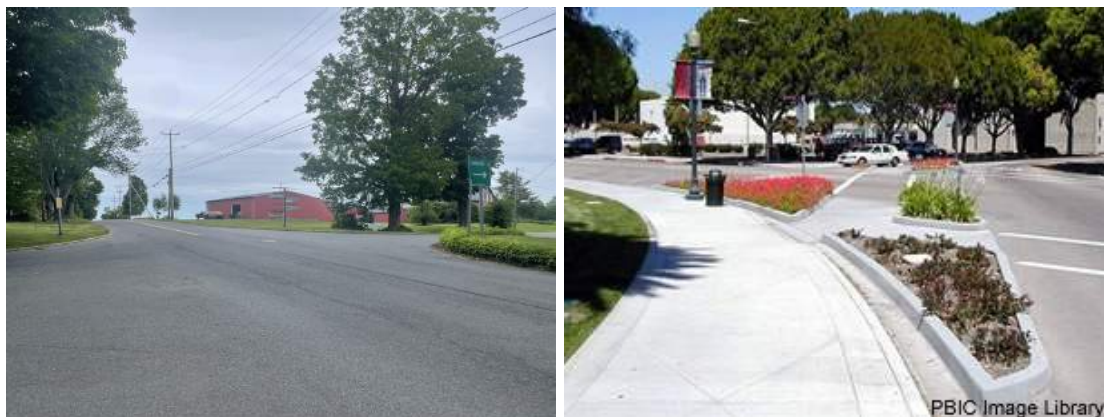
(Left) Wide curb radii currently at the intersection (Right): Reduced curb radii example from Safe Routes to School
