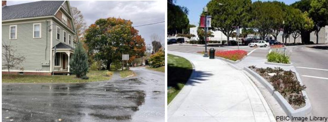
(Left) Wide curb radii currently at the intersection (Right): Reduced curb radii example from Safe Routes to School
