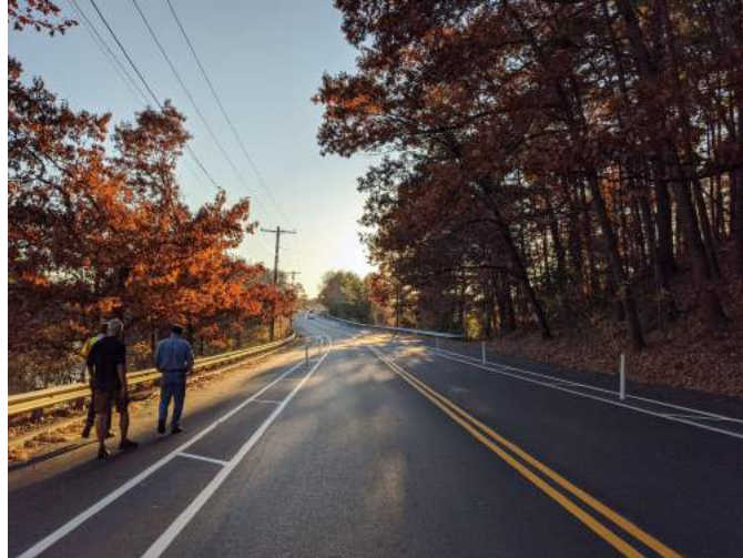
Flex-post protected walkway in Natick, MA
