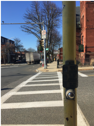
The pedestrian signals on Main St need to be replaced with updated Accessible Pedestrian Signals with countdown WALK signals
