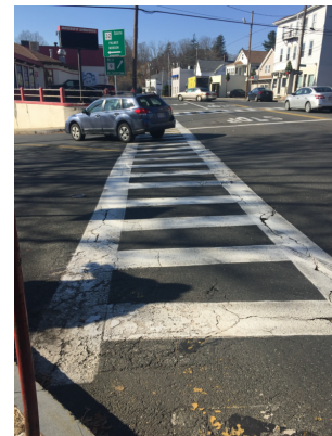
Poor sight lanes, vehicle turning patterns, and a long crossing distance at the Main Street and SR-32 intersection contribute to an unsafe walking environment in this location
