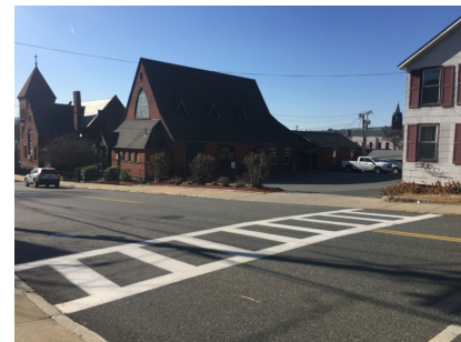
The midblock crosswalk to access the library on Church Street lacks features that make it visible to drivers
