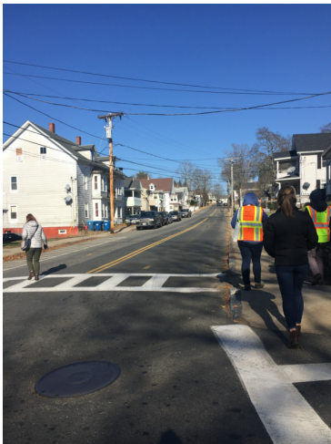
The intersection of North St and Pleasant St is traveled at high speeds and lacks advance pedestrian crossing signage
