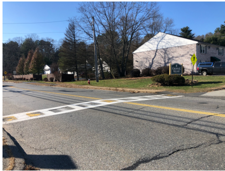
The safety of the midblock crossing at Colonial Village apartments could be enhanced with an RRFB
