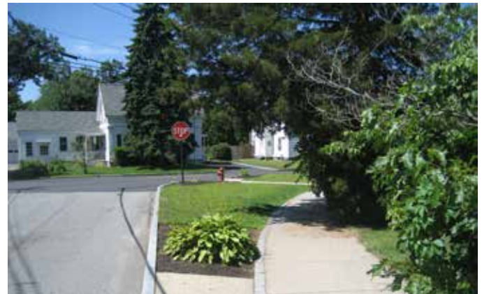
(B) Grass, trees and extended sidewalk in curb extension
