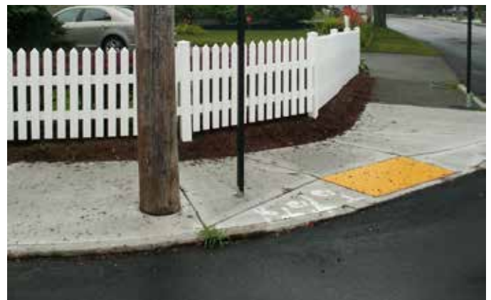
Curb ramp and detectable warning strip
