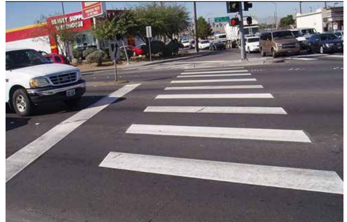
Crosswalk and stop line Source: http://safety.fhwa.dot.gov/ped_bike/tools_solve/ped_scdproj/sys_impact_rpt/images/fig16.jpg
