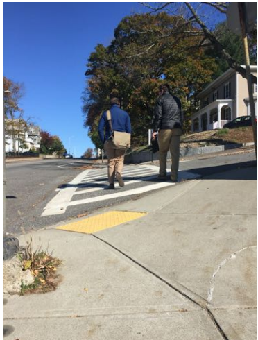
Crosswalks are steeply sloped on the hilly Lincoln Street terrain
