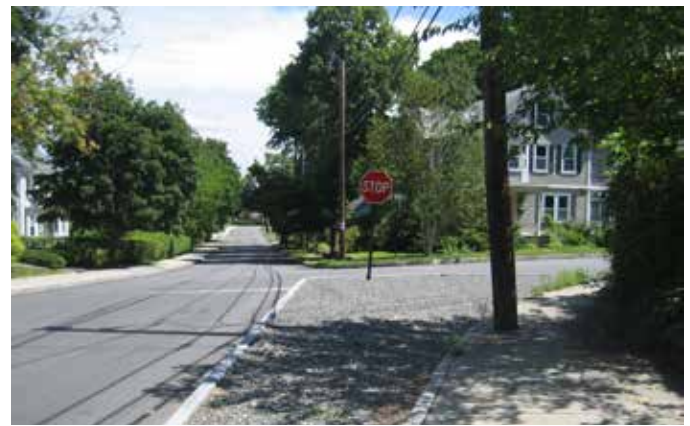
(A) Gravel-filled curb extension
