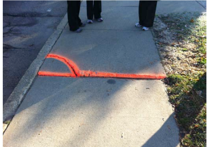
Large cracks in the sidewalk on West Central Street have been highlighted with paint, but not fixed.
