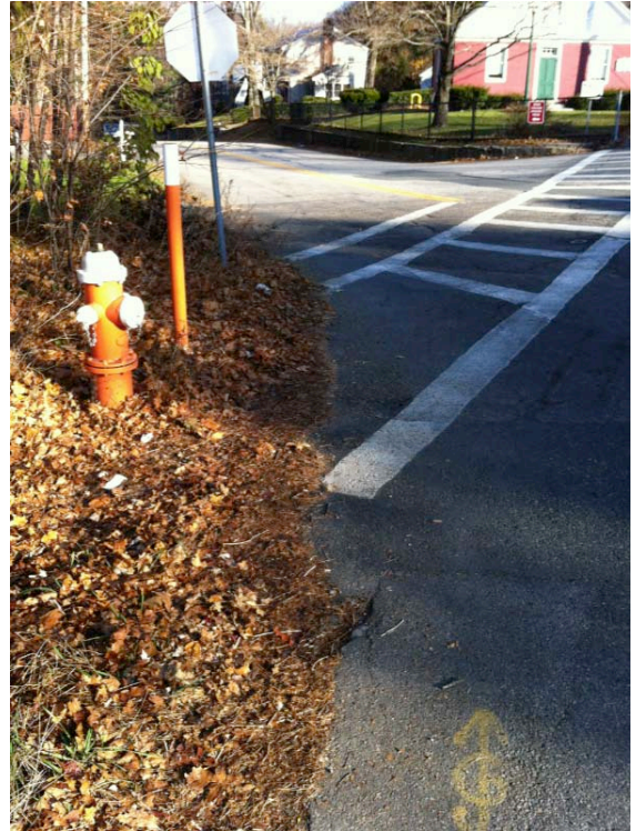
The crosswalk at Main and Maple leads into a hydrant and an unpaved shoulder.
