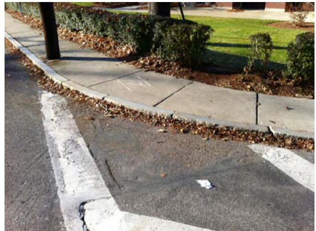
The crosswalk at Main and Church lacks accessible curb ramps.
