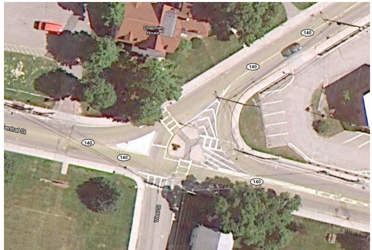
The intersection at West Central and Emmons requires pedestrians to cross multiple travel lanes and doesn't adequately slow traffic entering the school zone near Davis Thayer Elementary.
