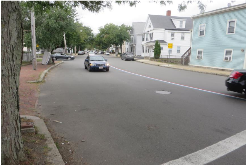
Excessively wide vehicular travel lanes lead to high traffic speeds on Washington Street.
