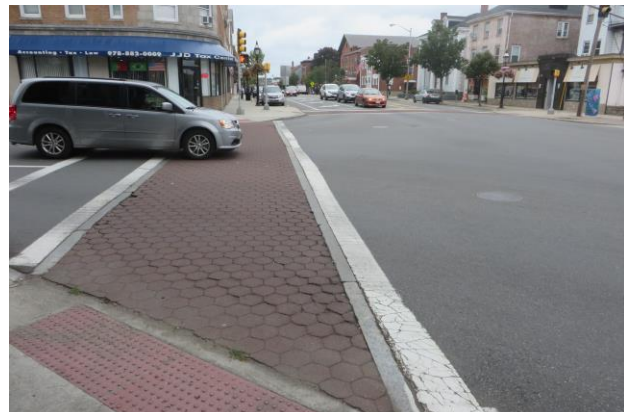
Bumpouts and refuge islands can help reduce long crossing distances at Main Street and Washington Street.
