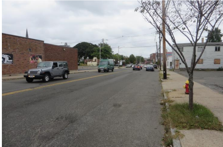
Excessively wide vehicular travel lanes lead to high traffic speeds on Foster Street.
