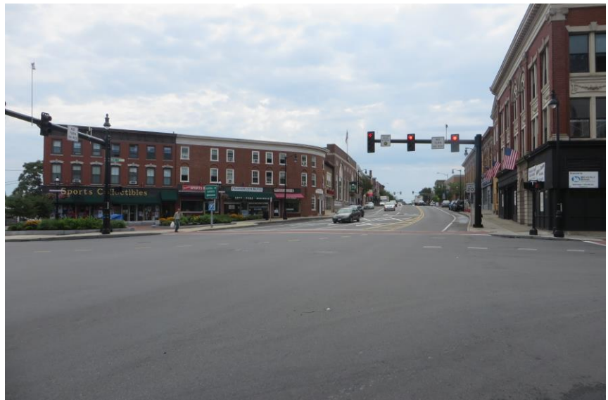
Long crossing distances, fast-moving traffic, and long waits for WALK signals pose challenges for pedestrians at the intersection of Main Street/Foster Street and Central Street/Lowell Street.
