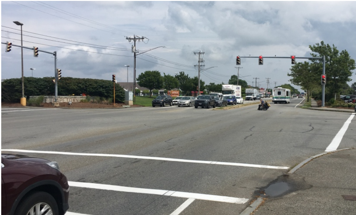
After navigating up the hill from the Cape Cod mall on the entrance road, this man in his wheelchair crossed Route 132 outside the crosswalk and proceeded up the Capetown Plaza entrance road within the travelway since no sidewalk was available.
