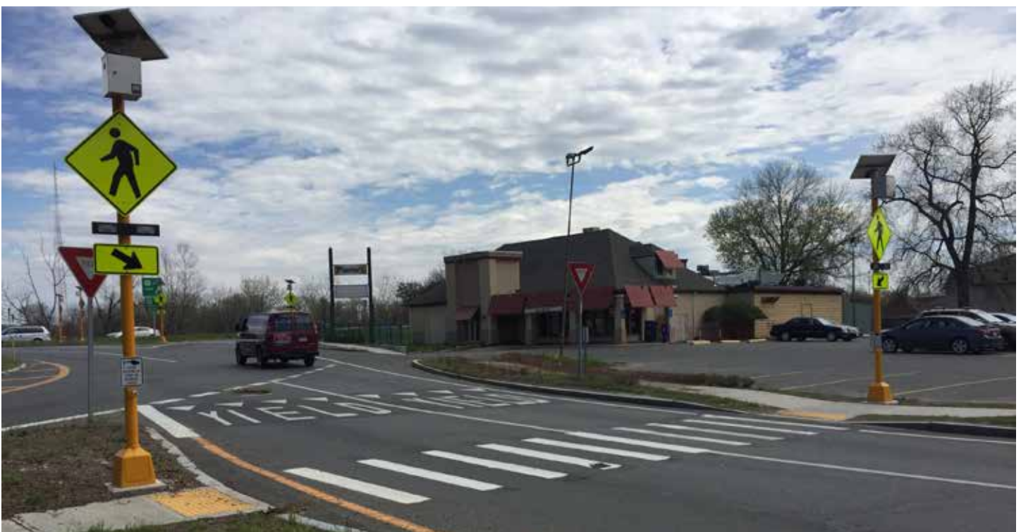
Rectangular Rapid Flash Beacons installed at the rotary are within 100' of the traffic signal and may pose a danger to pedestrians.
