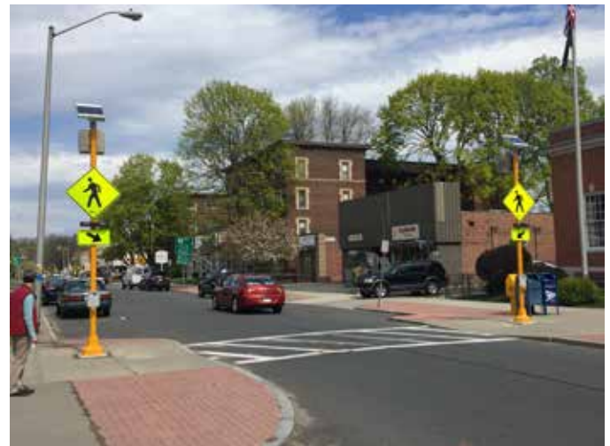
The crosswalk in front of the US Post Office on Elm Street has a Rectangular Rapid Flash Beacon and curb bump-outs.
