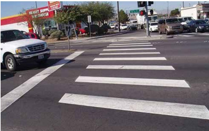
Crosswalk and stop line Source: http://safety.fhwa.dot.gov/ped_bike/tools_solve/ped_scdproj//images/fig16.jpg
