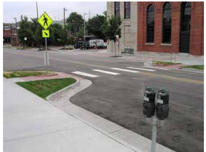
Curb extensions are often associated with mid-block crossings
