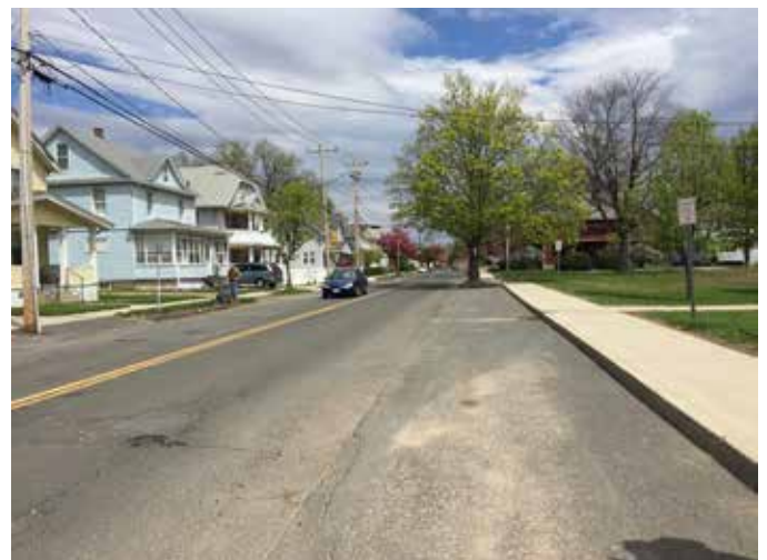
Drop off and pick up zone along Southworth Street
