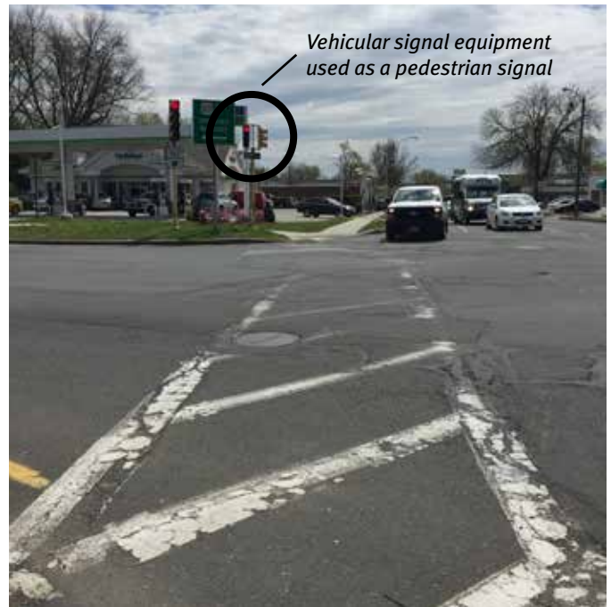
Park Avenue and Union Street intersection with long crossing distances and confusing pedestrian signal equipment
