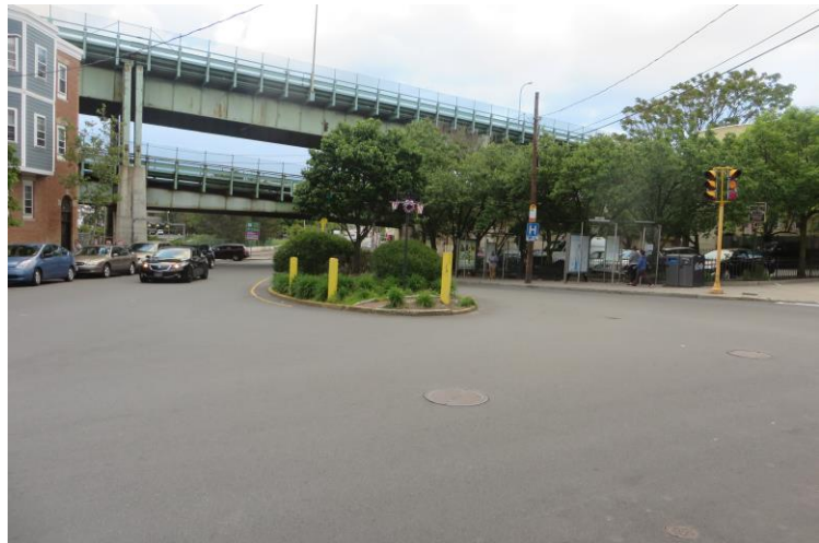
Wide travel lanes, nonexistent lane markings, and a missing crosswalk all present safety hazards at the intersection of Everett Avenue, Chestnut Street and Third Street.
