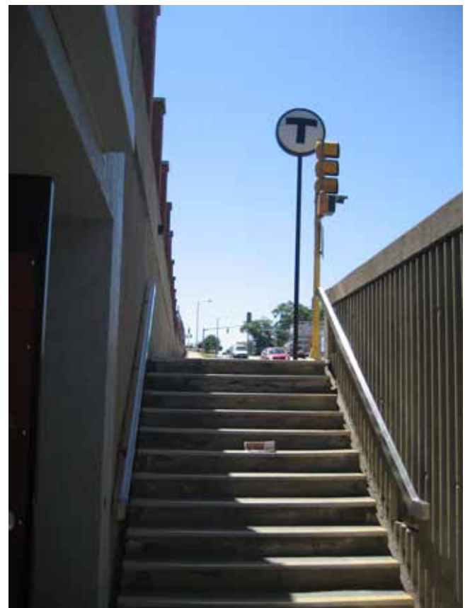
Accessibility is the focus of the MBTA effort to re-design Wollaston Station
