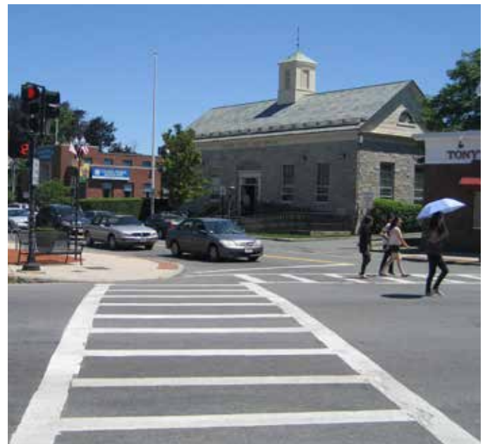
Crosswalks, curb ramps and pedestrian signals on Hancock Street
