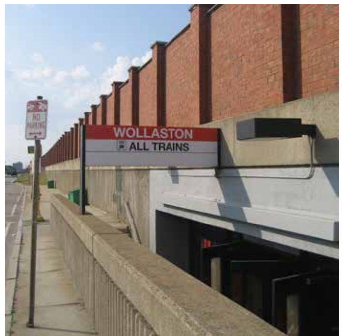
Wollaston signs face Newport Avenue, but there are none facing Brook Street. The sidewalk is narrow and has multiple obstructions which further limit its effective width. In the distance, the sidewalk ends providing no means of access for pedestrians.
