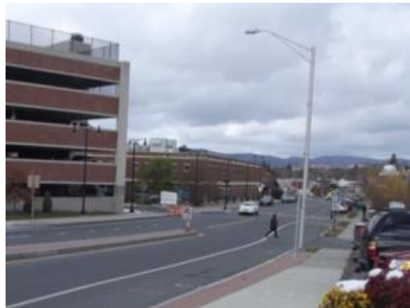
Figure 10: Pedestrian crossing intersection of Wahconah Street/Park Street on the south side of the intersection where the crosswalk was removed.
