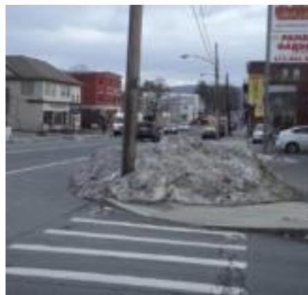
Figure 1: Curb ramp and sidewalk with snow.
