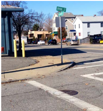
Figure 3: Apex curb ramp.
