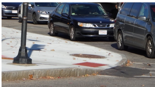
Figure 9: New curb ramp at the intersection of Mount Auburn Street and Common Street.
