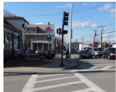
Figure 6: Apex curb ramp and pushbutton location at the Irving Street and Arsenal Street intersection.
