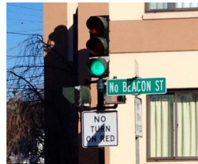
Figure 5: North Beacon Street name sign blocking the pedestrian indication.
