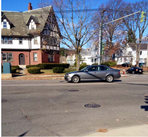
Figure 7: Missing crosswalk on the eastern side of Mount Auburn Street at Irving Street.
