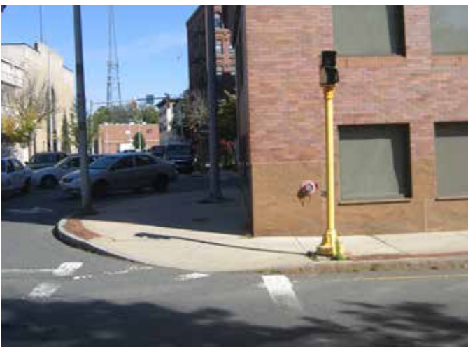
Broken pedestrian signal and faded crosswalks in Olympia Square
