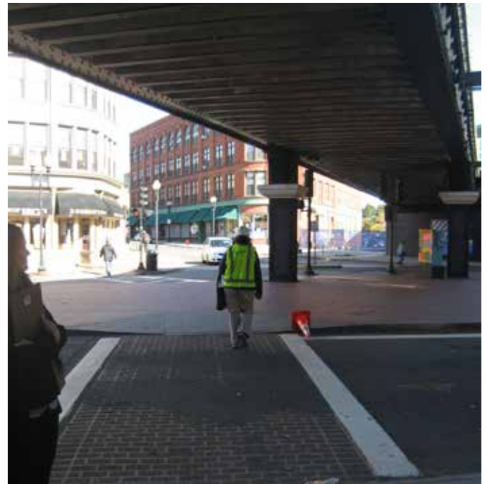
Crosswalk in shadow of overpass
