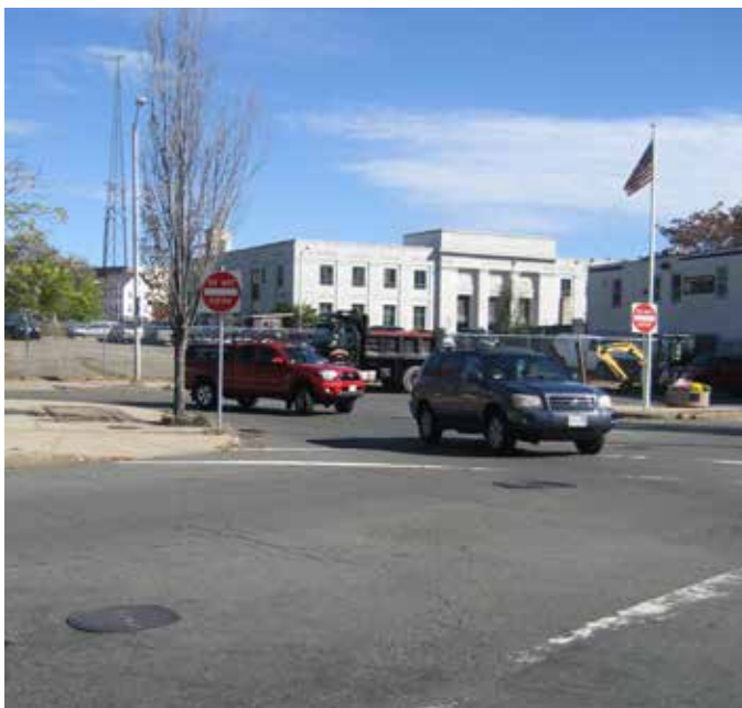
Faded crosswalks near the courthouse on Liberty Street
