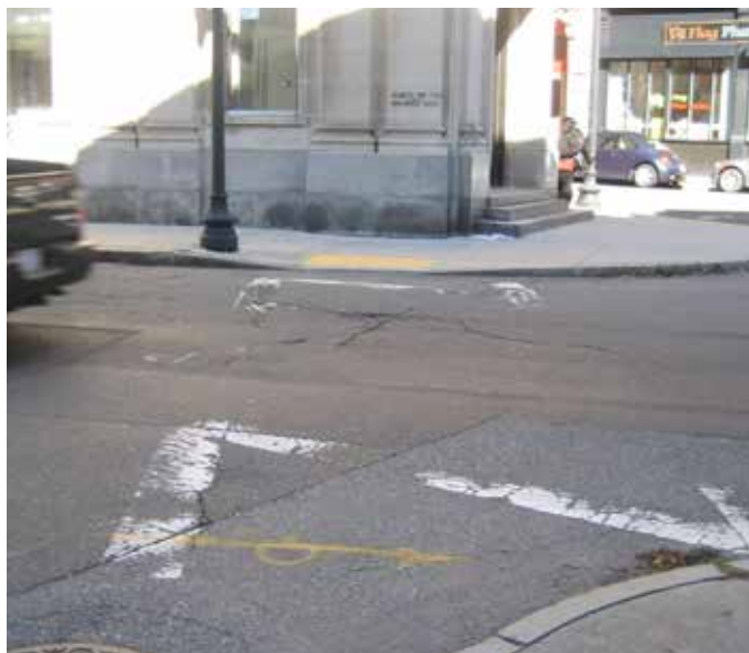
Faded crosswalk in Linnehan Square
