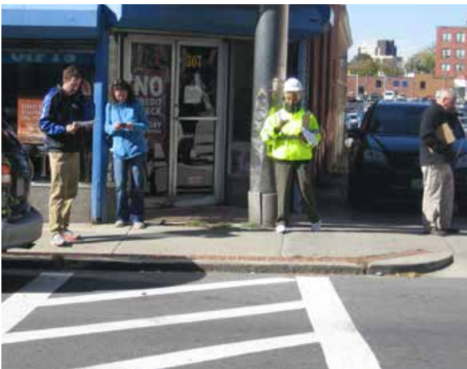
Missing curb ramp at the crosswalk on Union Street
