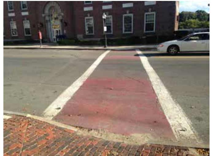
Mid-block crossing leading to the Post Office
