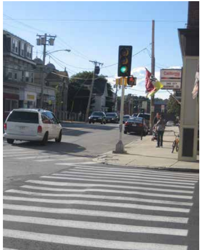
At the Winter/White intersection, the traffic signal obstructs the curb ramp; the sidewalk concrete has been damaged by turning trucks; and signal phasing does not prioritize the pedestrians
