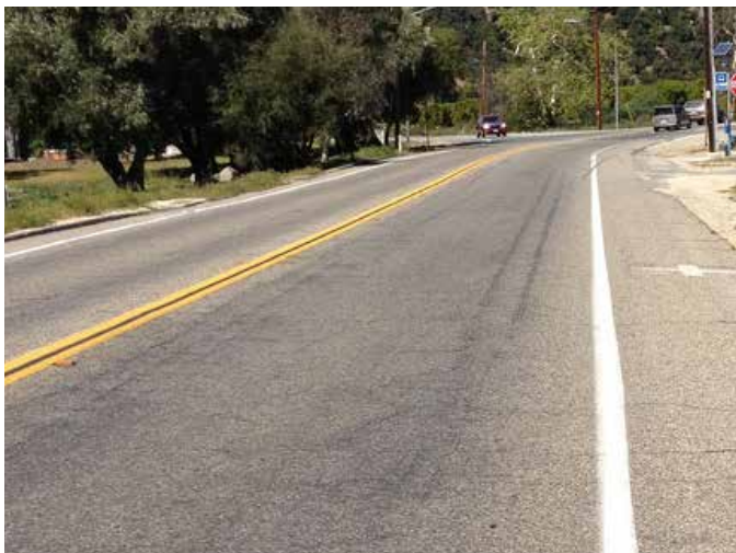
Edge lines delineate the vehicular driving zone on wide roadways.
