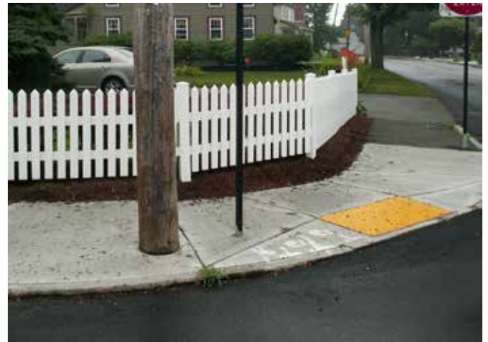
Curb ramp and detectable warning strip
