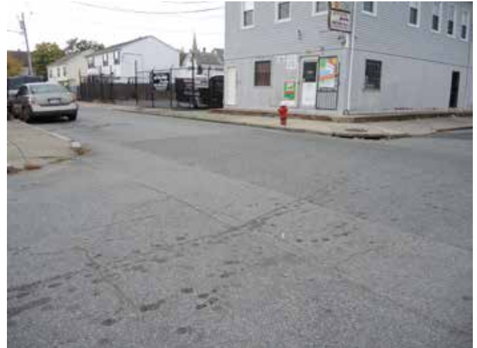
There are no marked crosswalks at the intersection of Grinnell Street and Acushnet Avenue despite the presence of a convenience store on the corner. Curb ramps and detectable warning panels are also missing.
