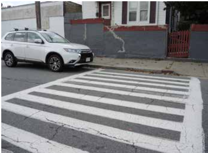
Cars parked directly adjacent to crosswalks block the view of oncoming traffic for people crossing
