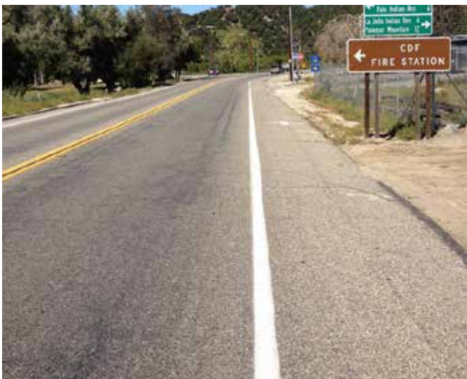
Fog lines delineate the vehicular driving zone on wide roadways.
