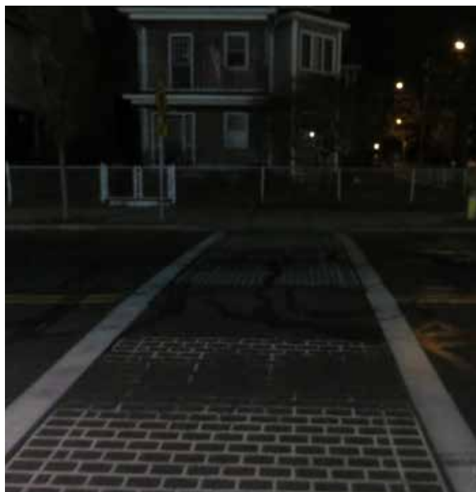
Crosswalk across Main Street near the Acushnet Avenue intersection
