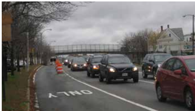
McGrath Highway, looking north
