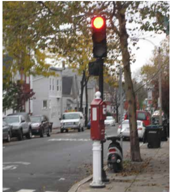
The pedestrian crossing signal is facing the wrong direction at the Cross/Pearl intersection
