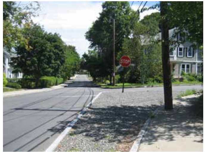
(A) Gravel-filled curb extension
