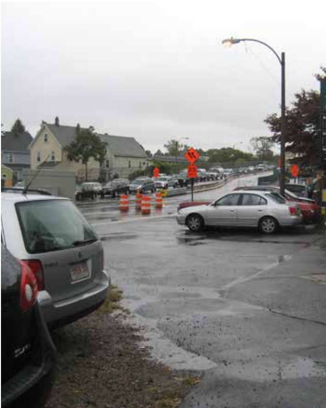
The parking lot of the auto repair shop on the southwest corner of McGrath Highway/Pearl Street intersection blends with the sidewalk compromising the pedestrian zone
