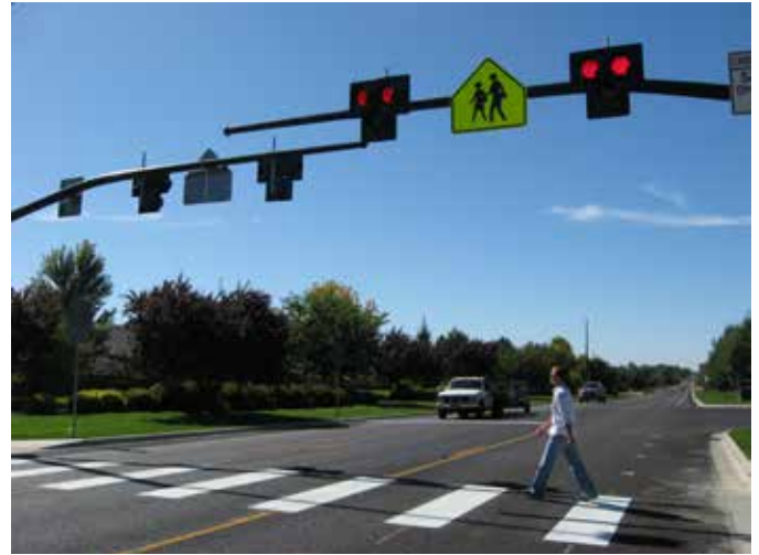
Walker crosses roadway after activating the HAWK beacon Source: http://www.achdidaho.org/Projects/Images/NewHawkSignal092209%20014.jpg
