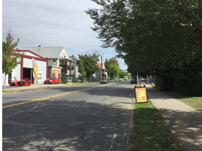
Carew Street corridor is a urban arterial with wide lanes and few pavement markings.
