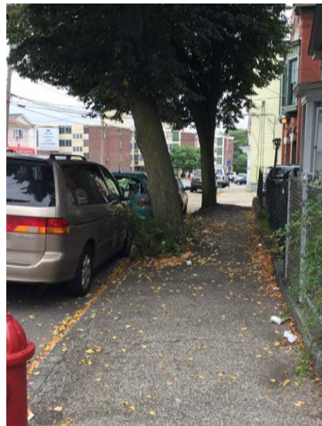
Trees along this sidewalk have made this section impassable for those with limited mobility or strollers
