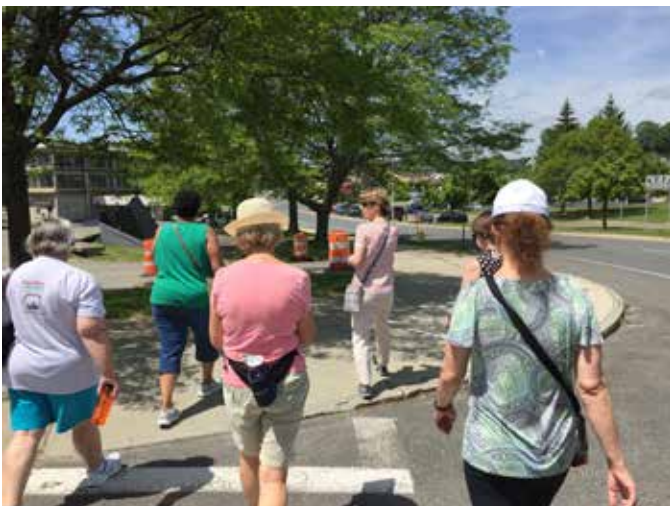
West Street has wide sidewalks and a buffer between moving traffic and the sidewalk. However, the sidewalks are in need of repair.
