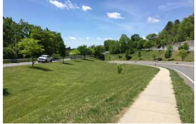
The sidewalk and buffer along Center Street are nice. However people attempt to walk along the road to the left in the picture, which has no sidewalk.
