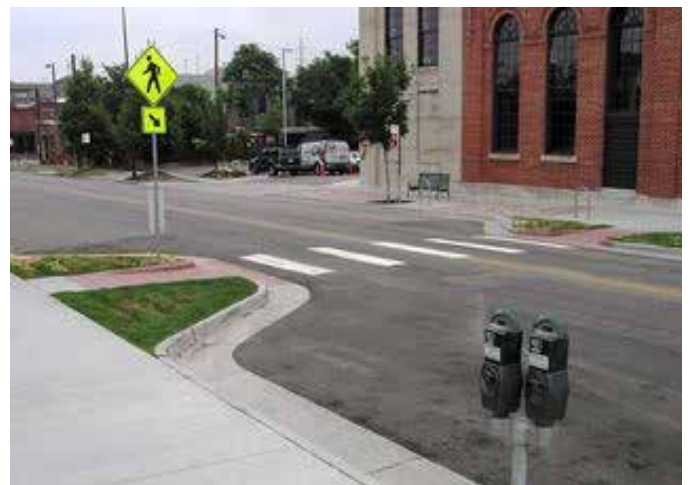
Curb extensions are often associated with mid-block crossings
