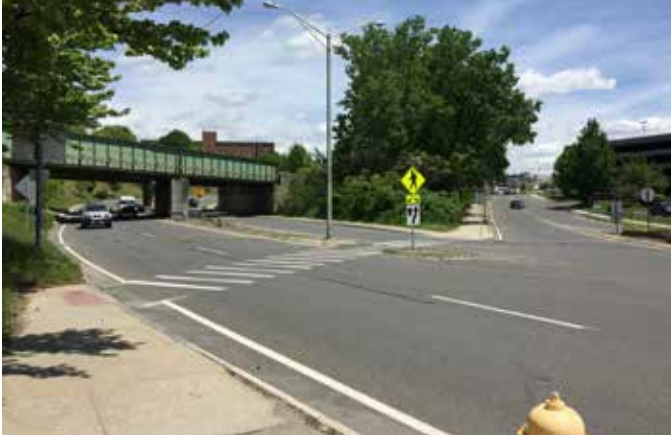
This crossing at Center Street can be dangerous given the high driving speeds and the changes in light drivers experience moving south beneath the overpass.
