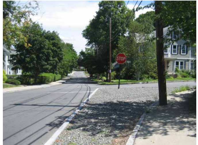
(A) Gravel-filled curb extension
