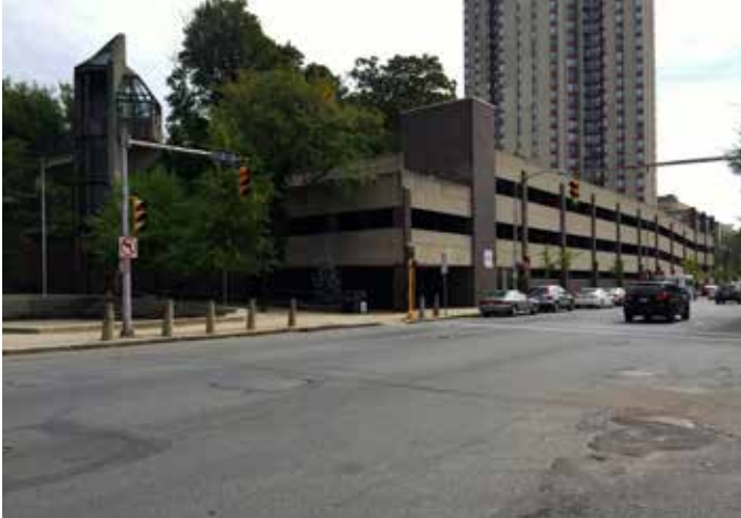
The Dwight Street crossing is long and not well-marked.
