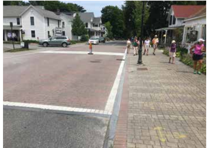
Ambiguous use of paving materials and flush curbs on Church Street
