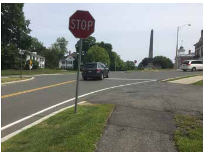
Views of Old Stockbridge Road approach where a crosswalk is needed. The sightlines, grade, and existing driveway make it more difficult to mark a safe crossing.
