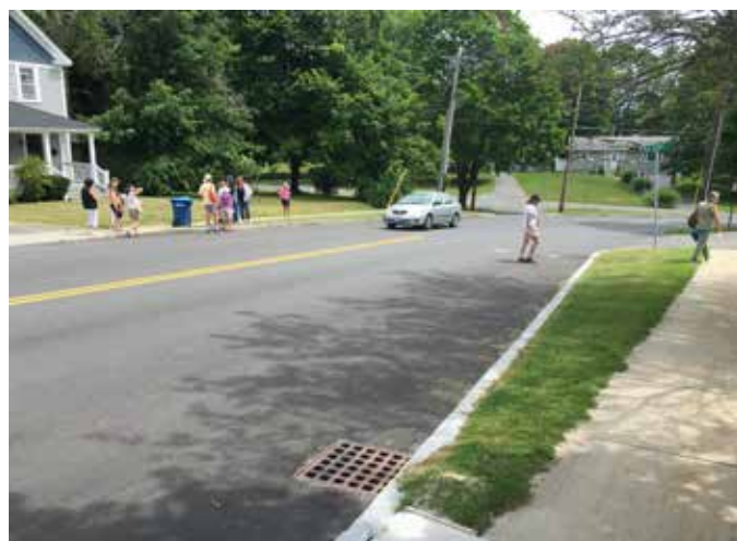
There is no safe place to cross between Ore Bed Park and the Community Center for many children who use both facilities.
