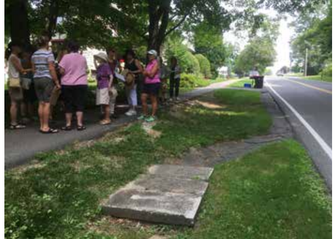
Asphalt sidewalks leading to the town center are in vary in quality and all are relatively narrow
