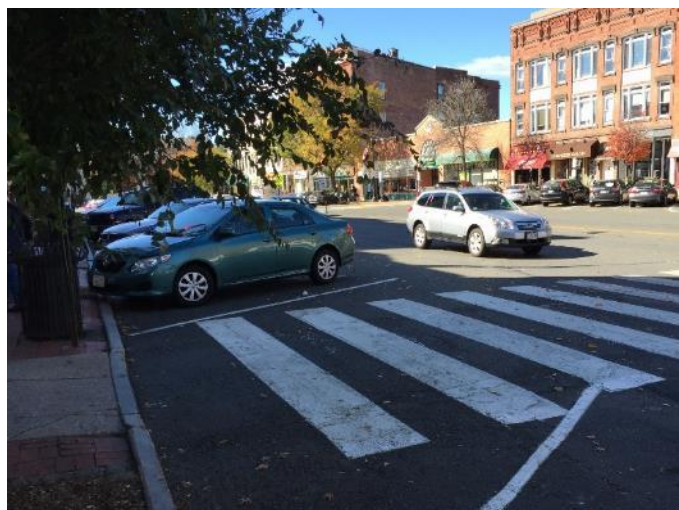
Figure 8 - Parked cars block sight distance to a midblock crosswalk.
