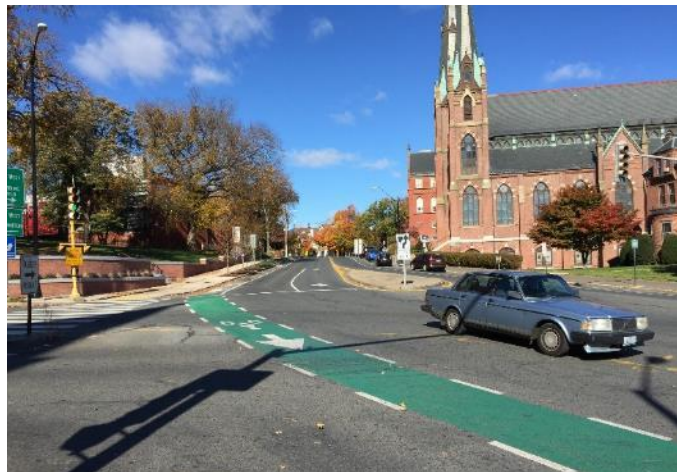
Figure 4 - Bike lane intersection markings transition through the West Street intersection.
