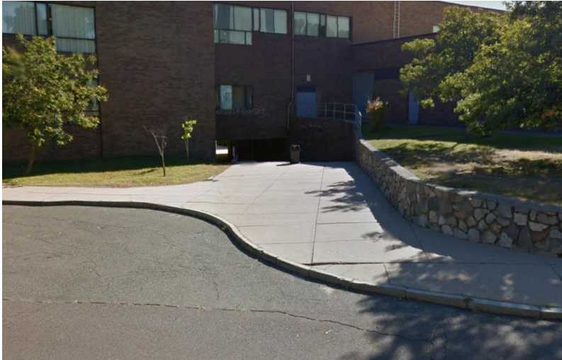
Underpass to courtyard is not bike-accessible
