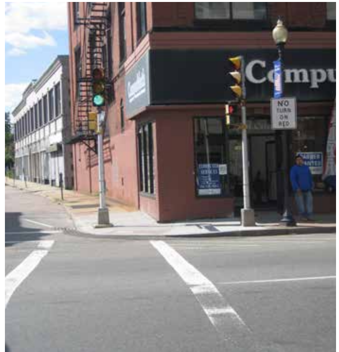
The pedestrian signal head is not lined up with the crosswalk entrance on N Main Street
