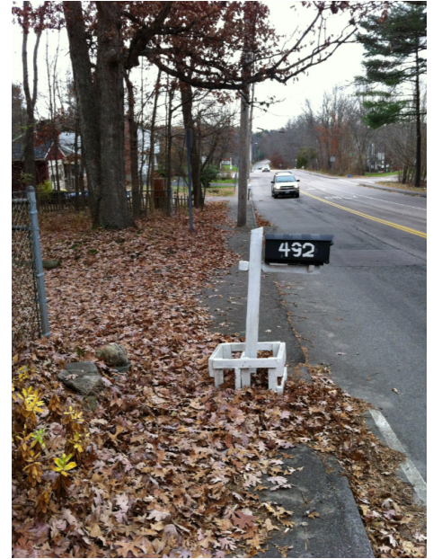
MAILBOXES SHOULD NOT OBSTRUCT THE SIDEWALK. THE TOWN SHOULD WORK WITH RESIDENTS TO FIND ANOTHER WAY TO MOUNT MAILBOXES THAT ALLOWS FOR SAFE PEDESTRIAN PASSAGE.
